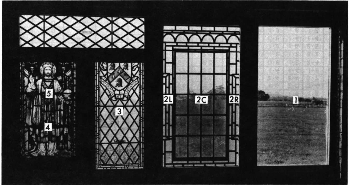
FIG. 10. Displacement transducer positions.
