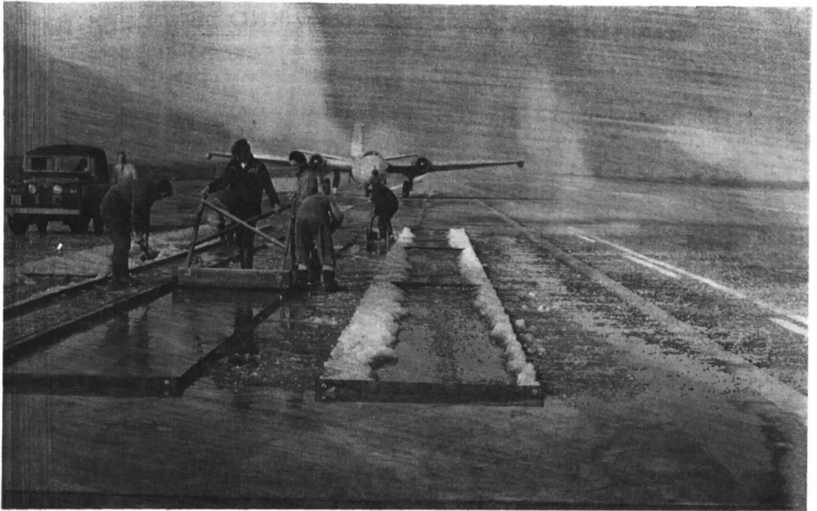
FIG. 11. Canberra wheel track in slush. One of the squeegees also shown in use.
