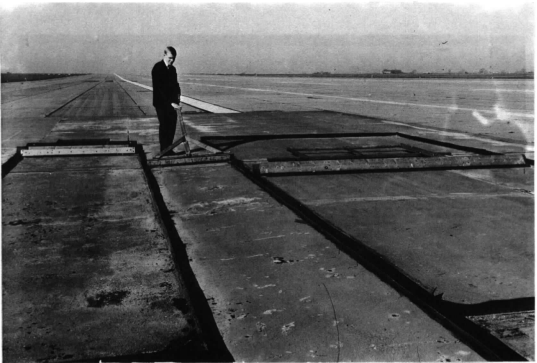
FIG. 5. Special squeegees for control of water.
